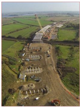
The main precast beams for the biggest viaduct to be built in West Sussex were delivered on 33 metre long vehicles with special police escorts.
