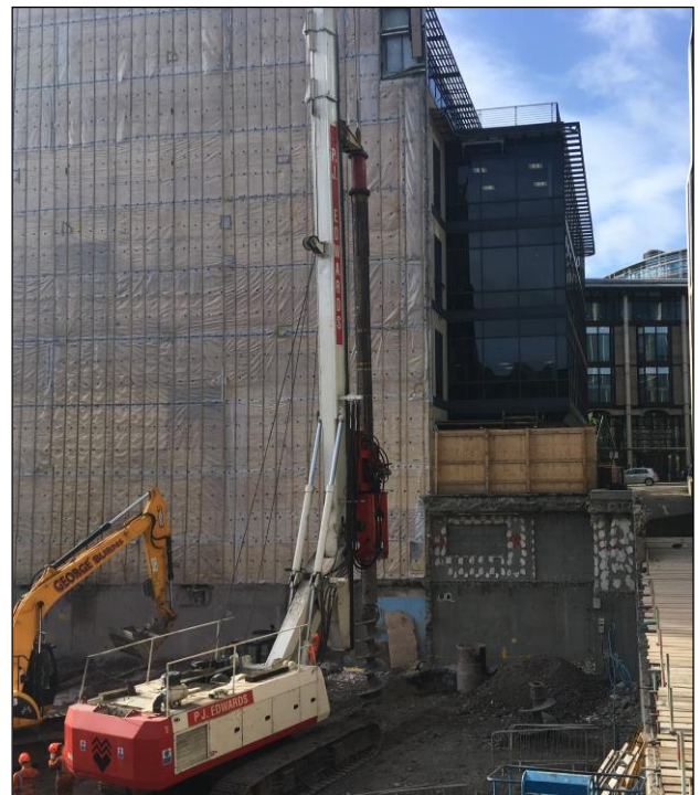
Mait HR260 piling rig installing contiguous bored wall piles
