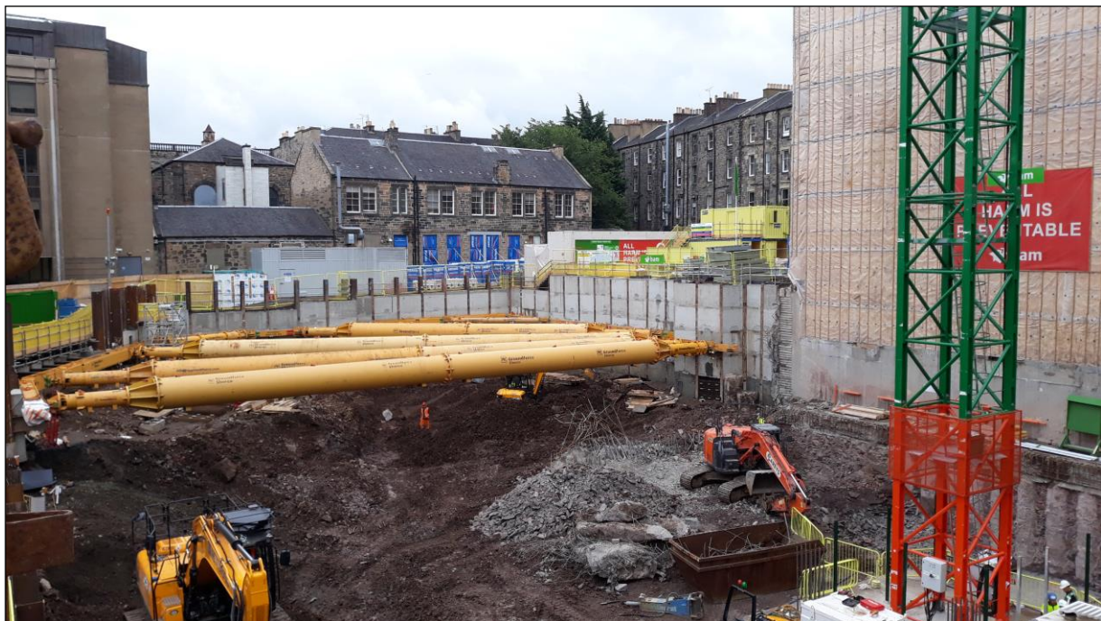
Kingpost retaining wall with support props installed
