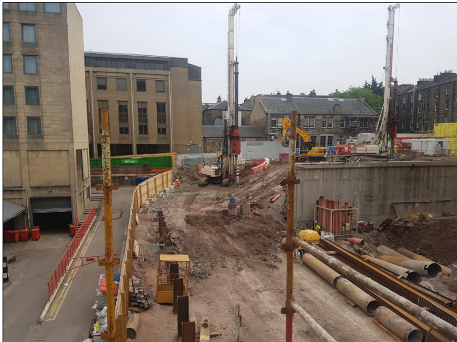
Installation of the bored kingpost wall
