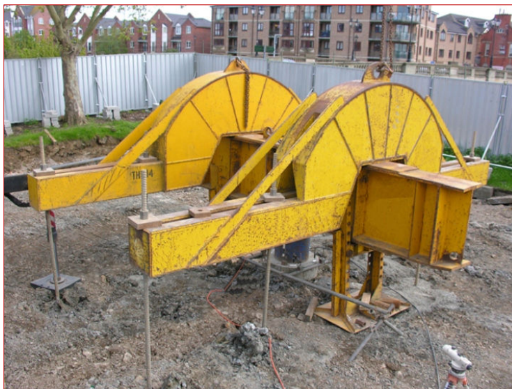
The 8 anchor pile load test at the Bottling Hall
