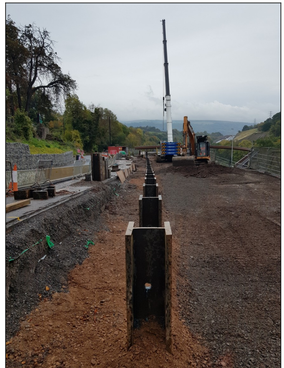
Installation of a kingpost retaining wall at RW31
