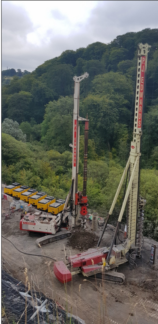
DTHH Piling at Retaining Wall RW14W
