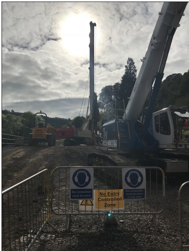
Installation of a kingpost retaining wall at RW31
