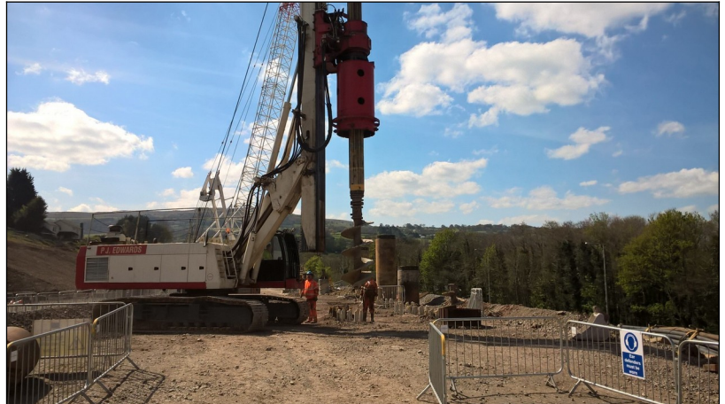
Traditional rotary piles being installed for foundations to Structure S11
