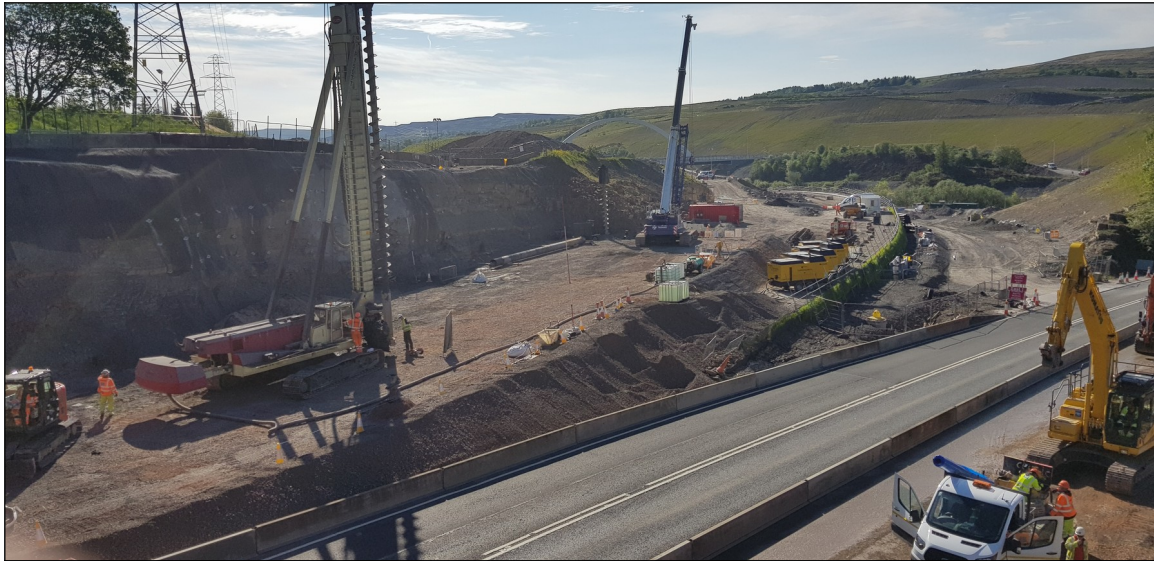
DTHH work at Retaining Wall RW02
