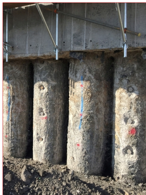
Details showing anchor bars and couplers to permit connections to basement lining walls and basement slab.
