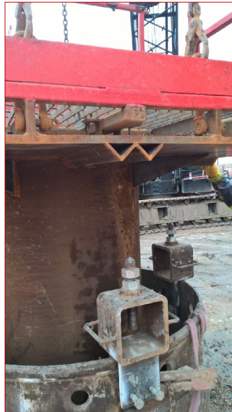
Guide Frame being lowered onto surveyed points on casing
