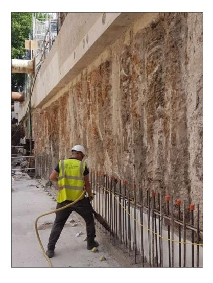
As the excavation progresses the excellent line of the secant wall can be seen and demonstrates our ability to install secant wall piles to the strict tolerances required.
